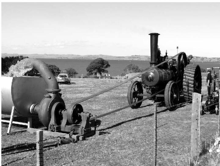
1907 Foden as Stationary Engine & Pump
